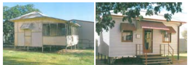
The Opera House Photographic Gallery, before and after restoration.
