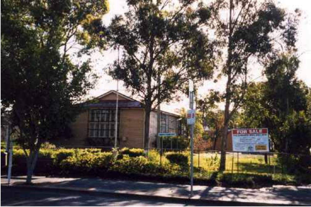
Sandgate Drill Hall
