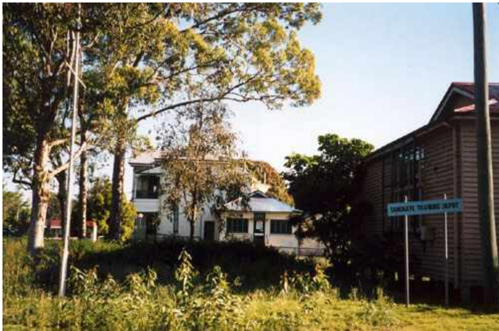
Sandgate Drill Hall looking towards the Post Office complex and railway station -far red roof. (September, 1999)
