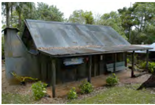
The Slab Cottage – constructed from genuine slabs recycled from other buildings. Typical of the lifestyle of the earliest settlers on Tamborine Mountain in the late 19 th and early 20 th centuries
