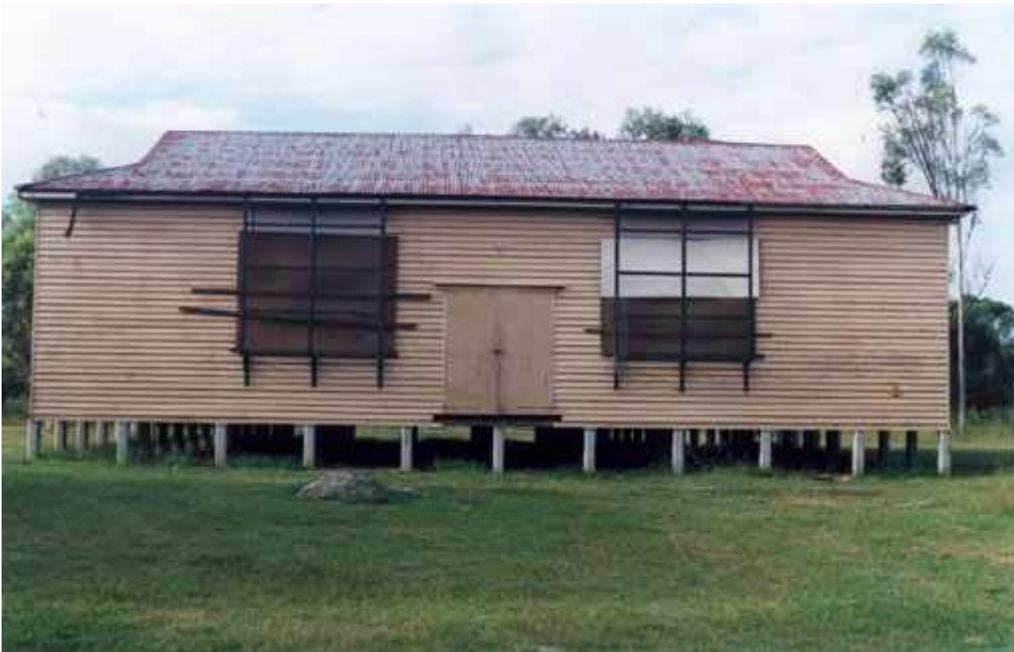
**Sandgate Drill Hall moved to its new site -note elevation and replacement concrete stumps (February 2000)**
